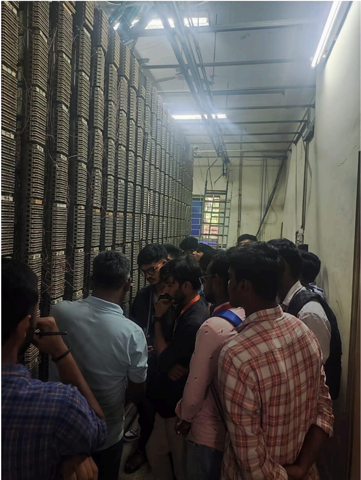
BSNL Expert explaining about Fault Tolerance of Copper Cable Connection of Telephone Systems
