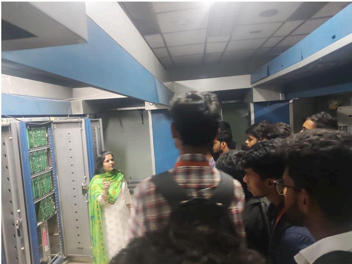
Mrs. Monika is discussing about CDOT used in Switching Systems
